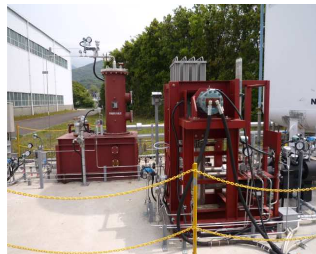
LNG High Pressure Pump, Heat Exchanger
