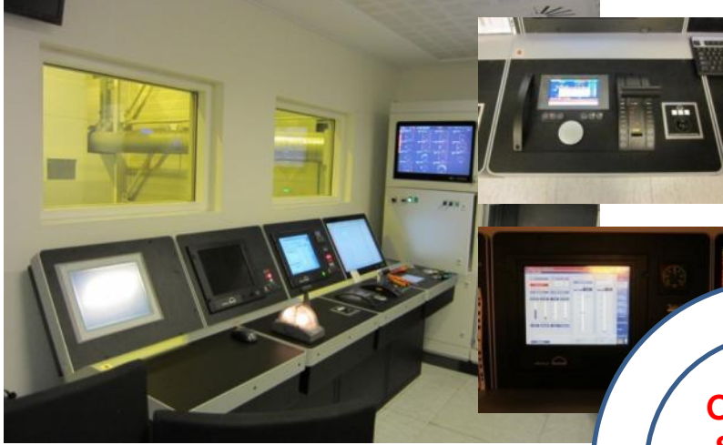
ENGINE CONTROL SITE
