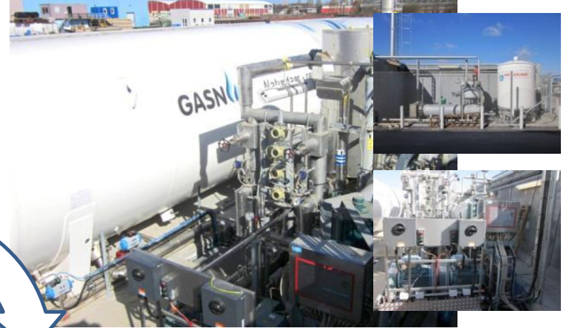
FGS SKID SITE
