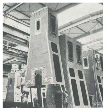
Fig. 53 Engine columns ready for assembly. (GV [3])
